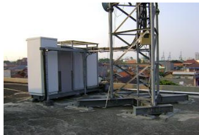
Gambar Rooftop Tower
